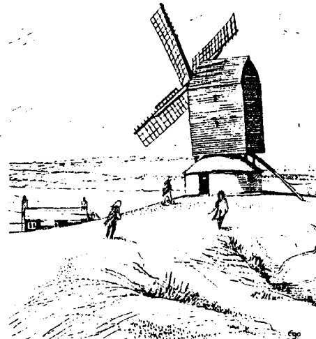
Brill's post mill. These old mills were mounted on a single post, and the whole body of the mill turned to bring the sails into the wind. Smock mills, like the one at New Bradwell, Milton Keynes came later. Only the bonnet, on a smock mill, turned with the sails.
